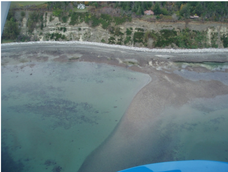
Photo 3: Continuous riprap along base of Willemar Bluffs, 2003
