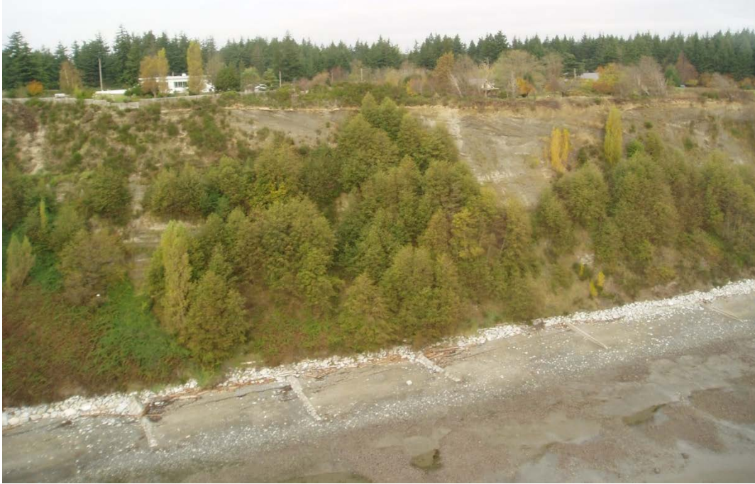
Photo 4: Groynes and riprap at southern end of Balmoral Beach, 2003
