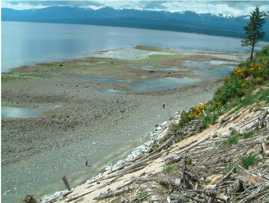
Photo 2: New riprap along base of Willemar Bluffs with tidal pools in background, May 2003
