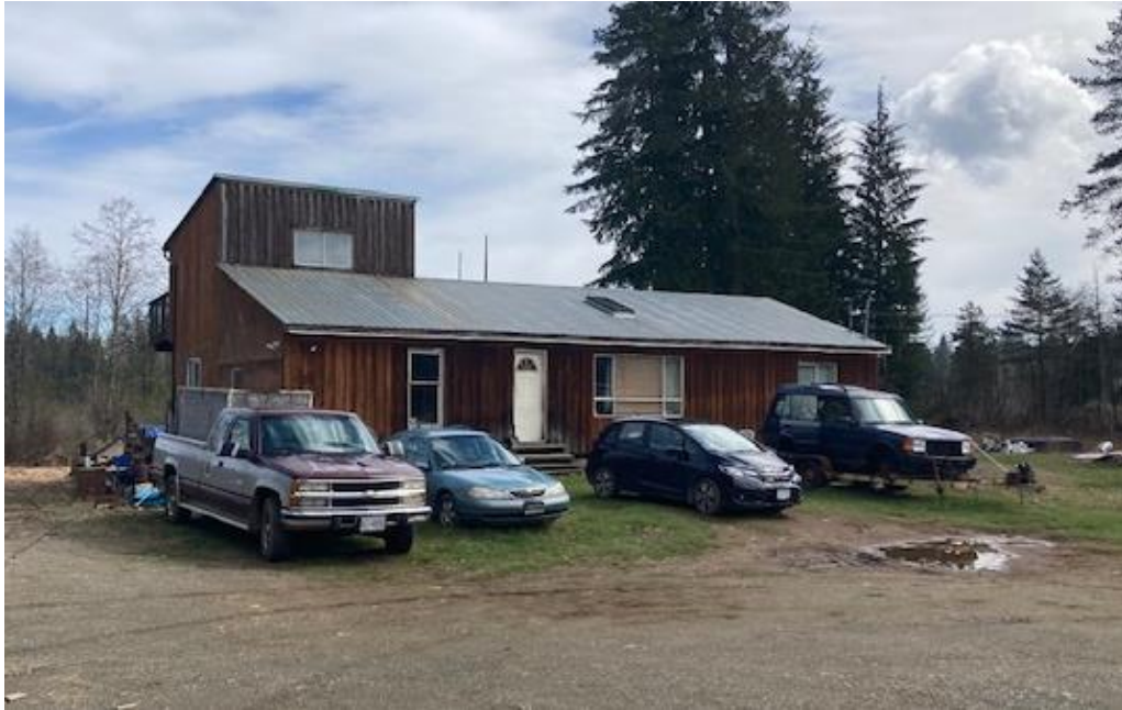
Photo 5: Exterior view of the secondary residence at the south end of the property.
