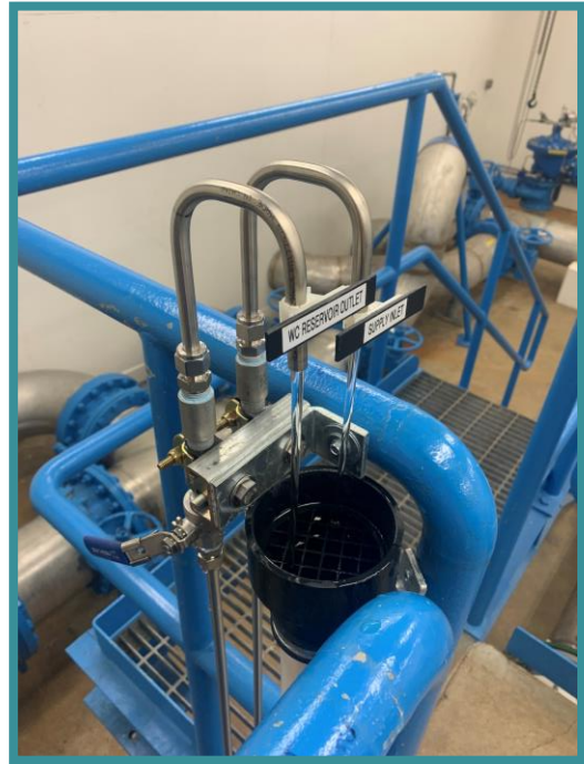
Sample taps at West Courtenay Reservoir.
