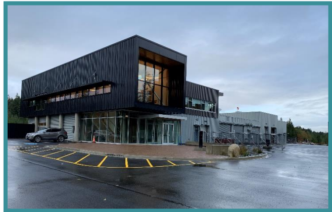
Comox Valley Water Treatment Plant
