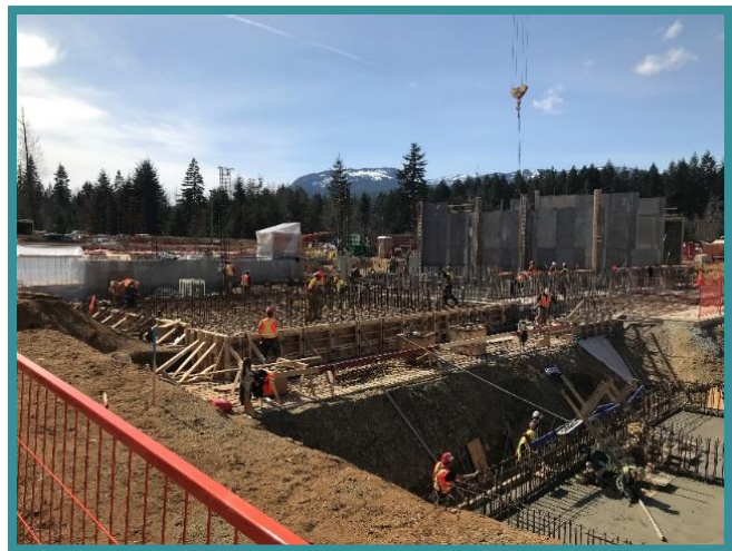
Construction of the water treatment plant in 2020.
