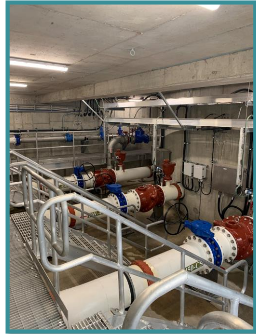
Pumps at the raw water wet well.
