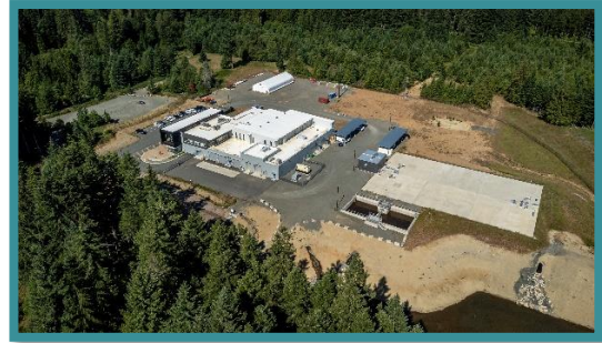
Above: Comox Valley Water Treatment Plant.
