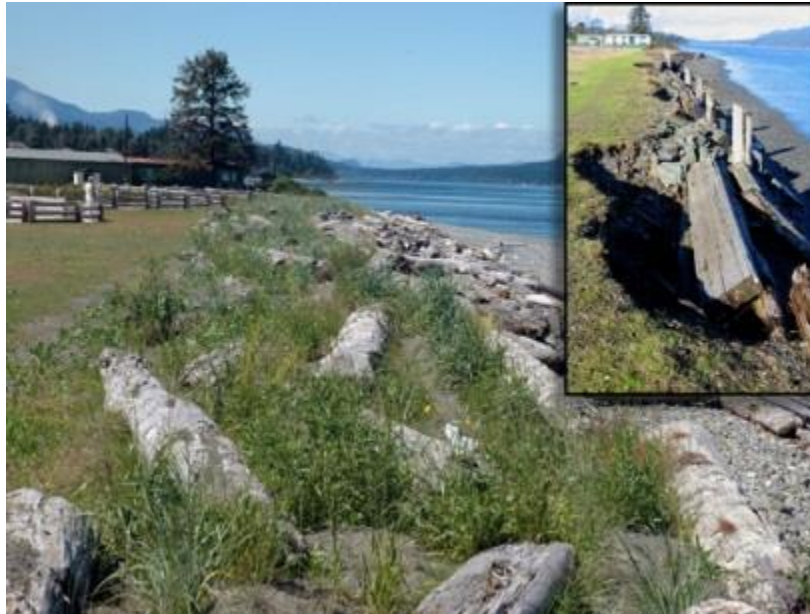
Above: Before and after beach nourishment (soft shore) at Tyee Spit, Campbell River Photo: B.C.P. Harrison
