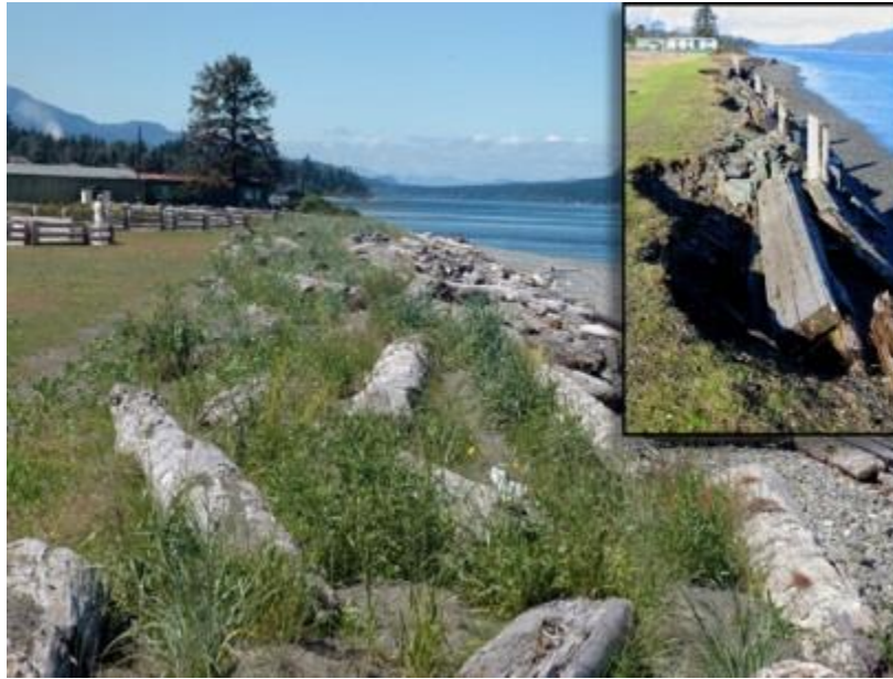
Above: Before and after beach nourishment (soft shore) at Tyee Spit, Campbell River Photo: B.C.P. Harrison
