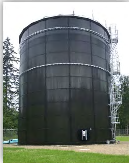
Treated Water Storage Reservoir 490 McLeod Road Top Water El. = 92 m
