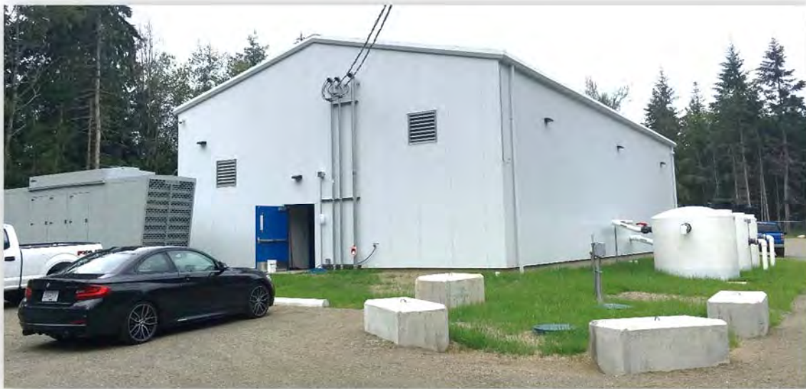
Water Treatment Plant Building, Exterior
