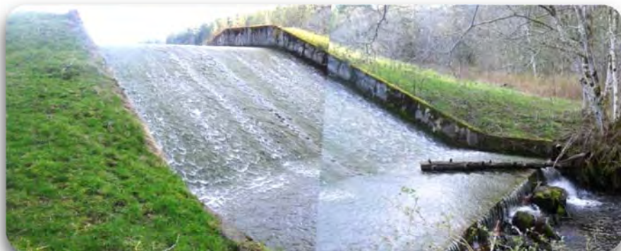
Langley Lake Outlet Spillway (Crest El. = 152.17 m) April 11, 2022
