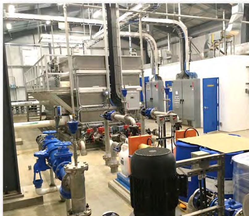
Water Treatment Plant Building, Interior
