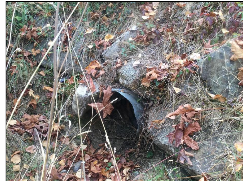
Unnamed ditch crossing
